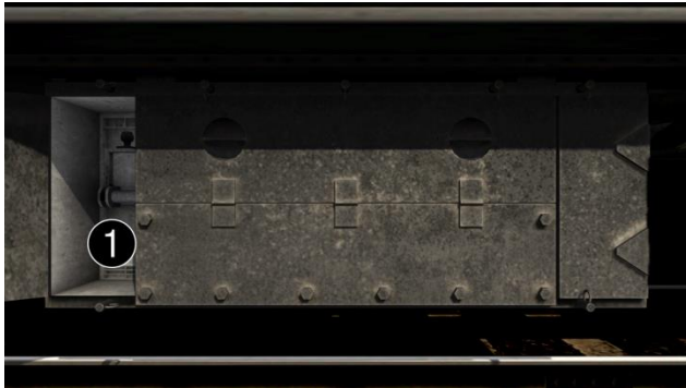
1 - Battery isolation switch (in/out)
