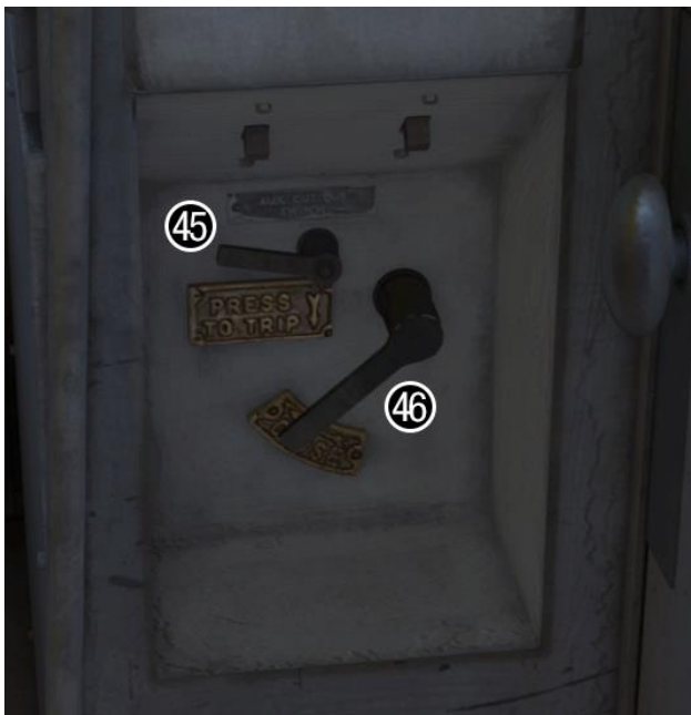
45 - Auxiliary Isolation Switch (AIS) TRIP 46 - Auxiliary Isolation Switch (AIS) CLOSE
